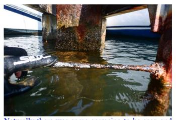
Naturally there was some corrosion to be seen and photographic records were made (above and below the surface) for future reference. As was to be expected, the corrosion was most apparent on the ladders in the early part of the estate. Since these were installed 30 years ago, they have done well. We have diarised the next survey for 2023.
